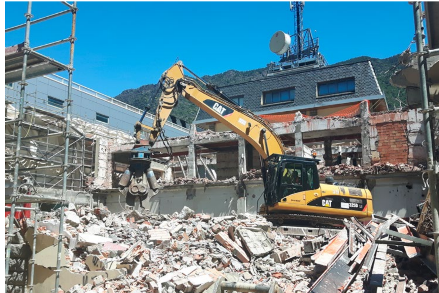
> Andorra Telecom building demolition
