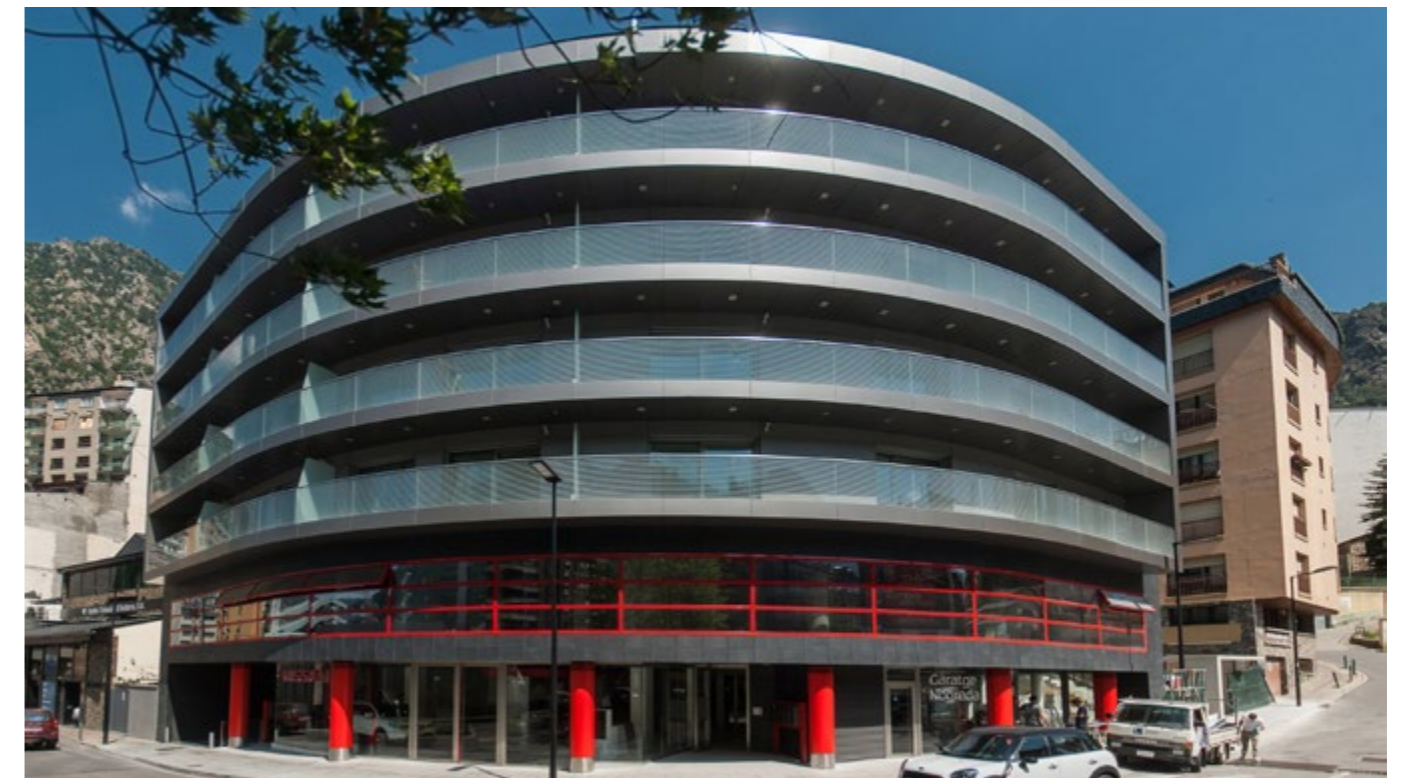
> La Quirota Building
