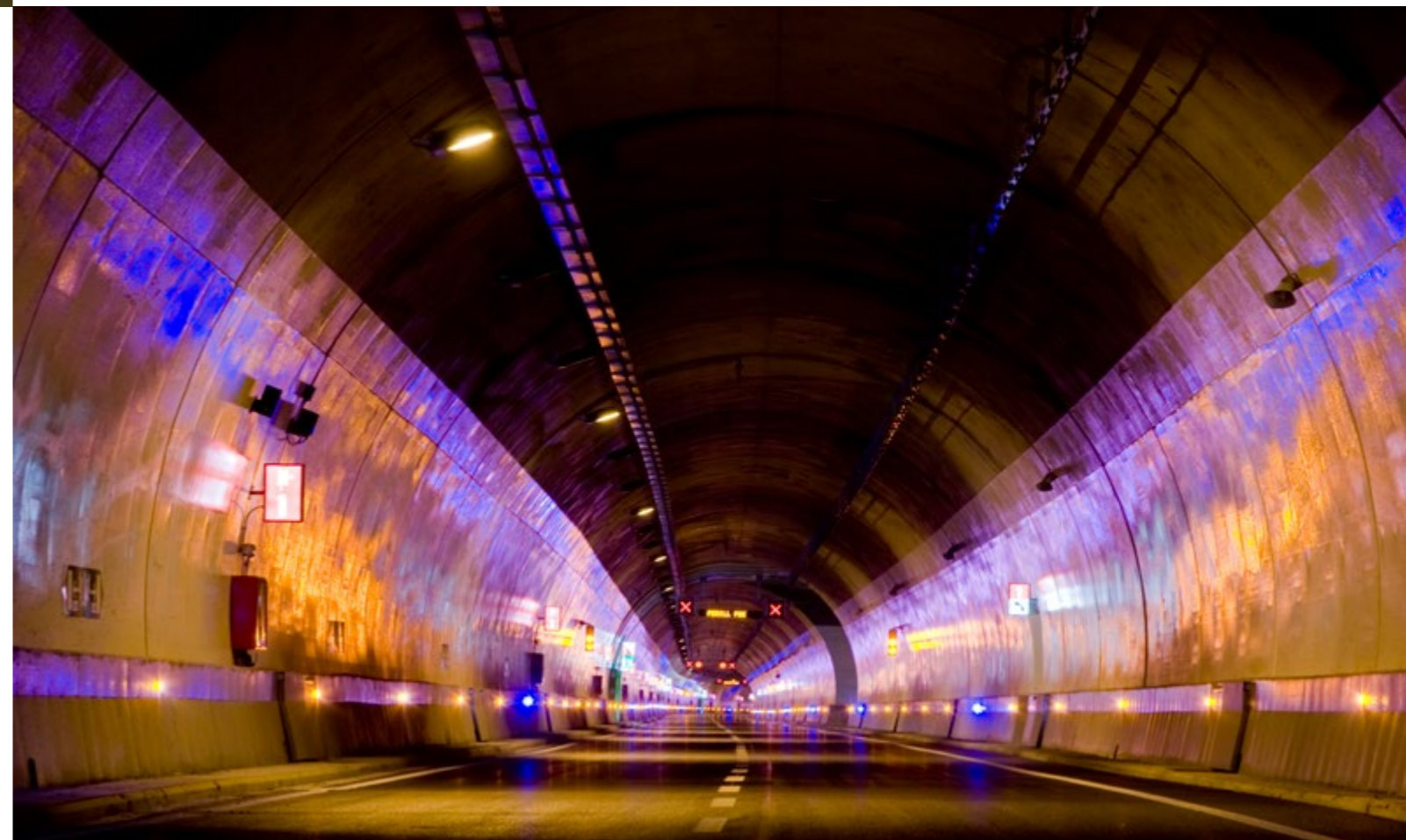
> Dos Valires tunnel
