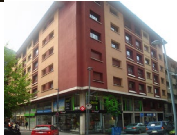
> Capri Building (before and after)
