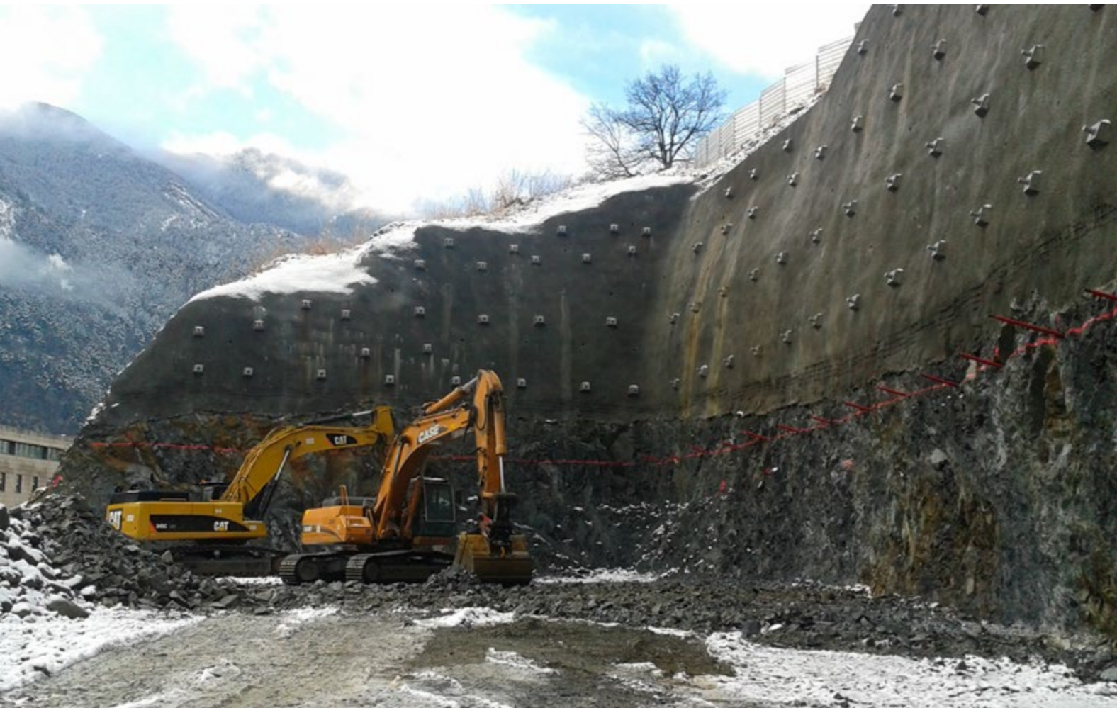
> Falgueró Car Park Excavation
