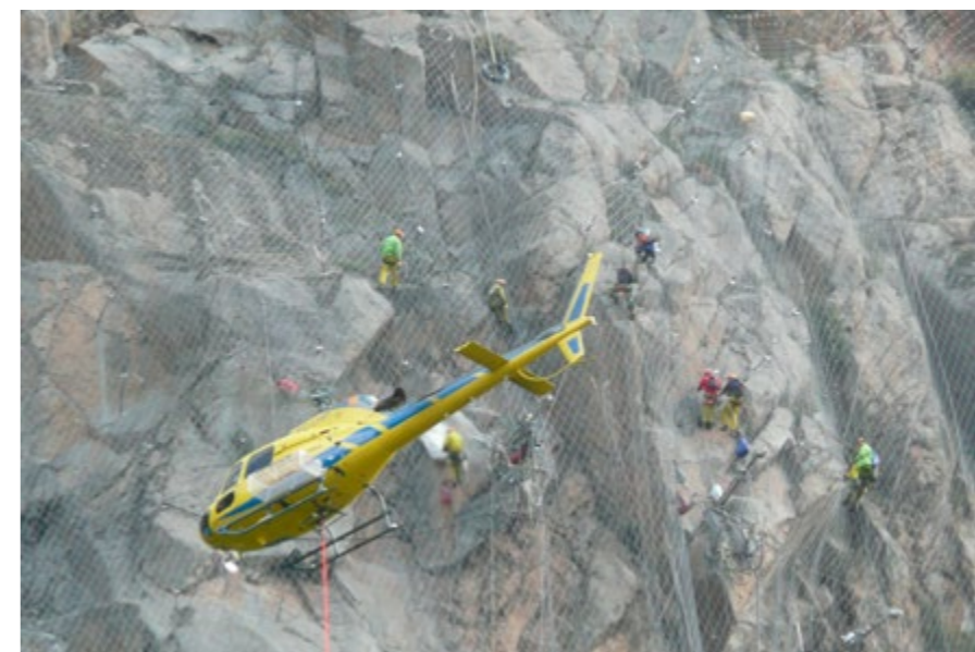
> Stabilisation of the Roc del Corb slopes
