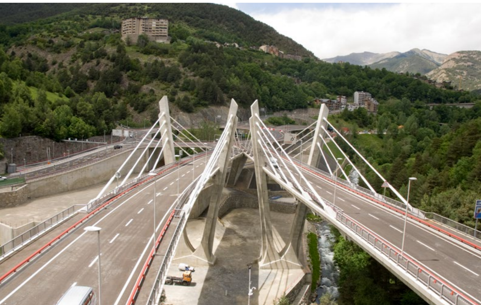
> Dos Valires Access Tunnel
