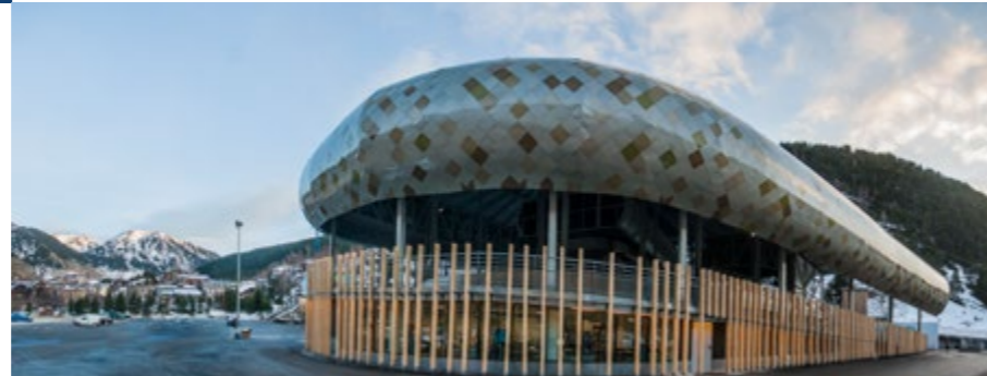
> Tarter Cable-Car Building
