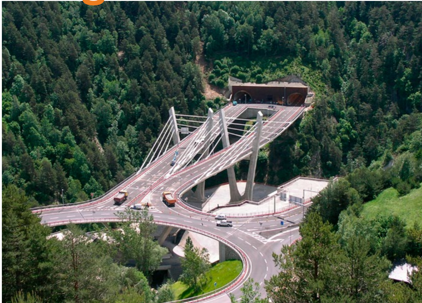
> Dos Valires Access Tunnel
